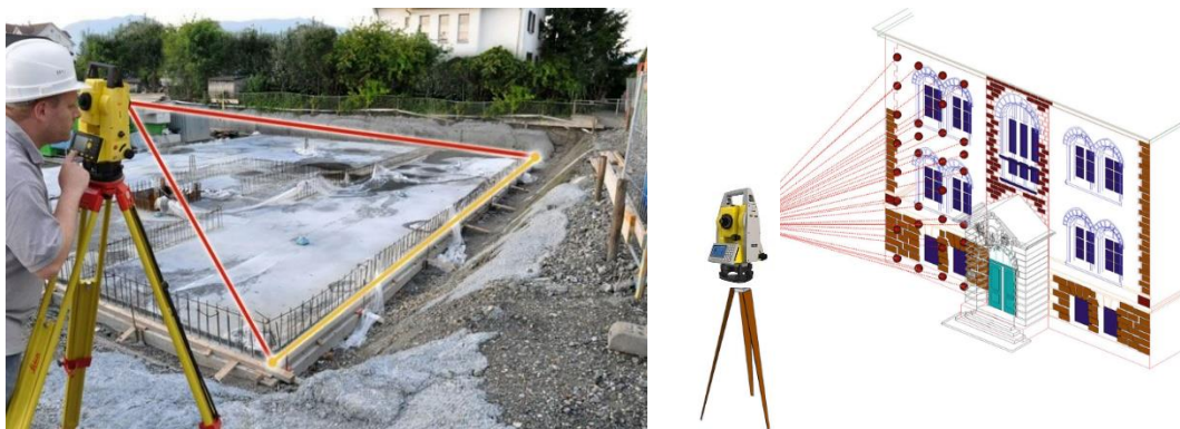
Figure 4. Staking out with tachymeter and As-built survey
